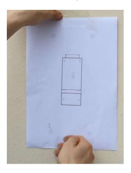
Stick the drawing on the wall with tape to decide the drilling hole position.
