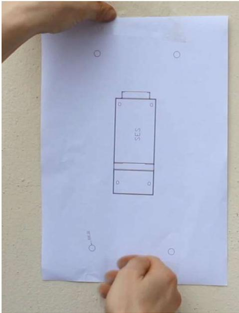
1. Stick the drawing on the wall with tape to decide the drilling hole position.
